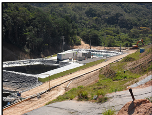
Figure 3. Leachate Treatment Station (LTS)
