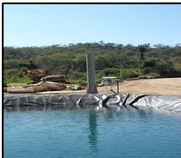
Figure 5. Treated Leachate Collection Pond
